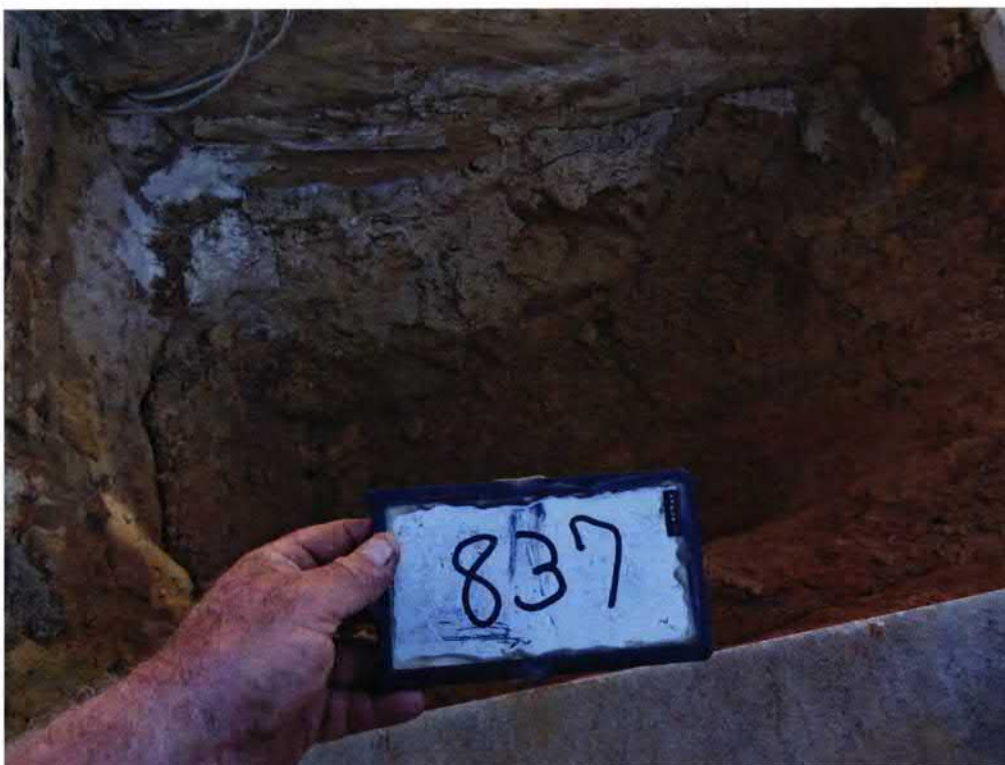
Picture 2: UST 837Azalea excavation.
